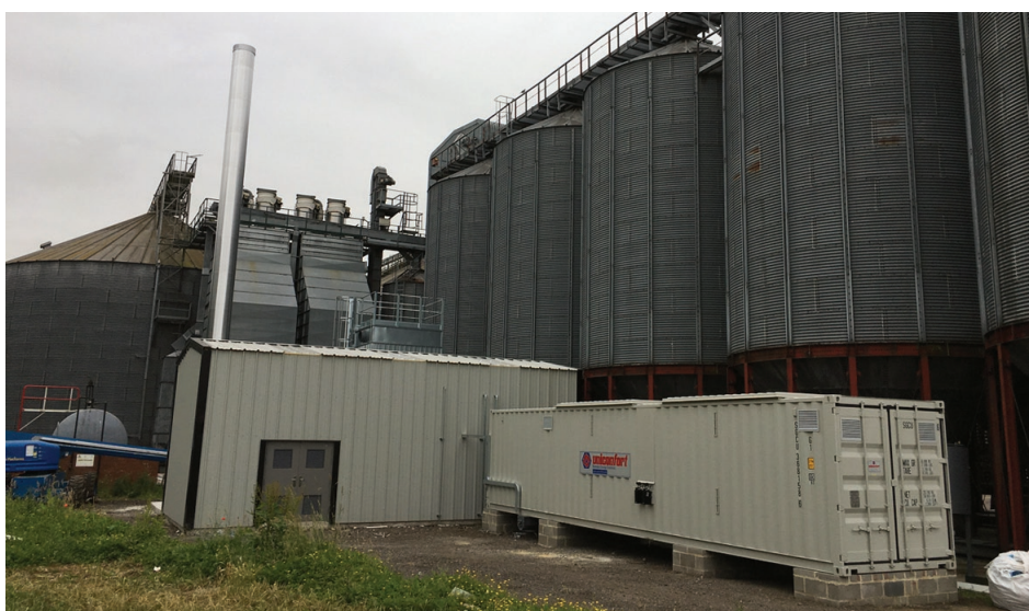
New bio-mass boiler at Piercebridge.
